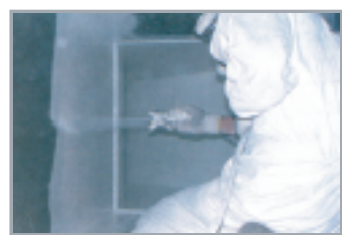
Applying an Anti-Microbial Treatment inside a Duct
